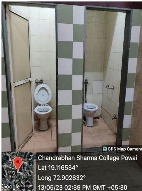
Washroom facility for Girl
